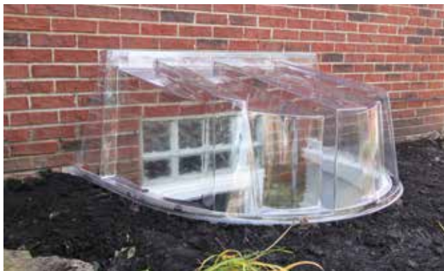
If the well is installed on an existing window, you must use a dome style cover, fence, or other enclosure to ensure safety around the well.
